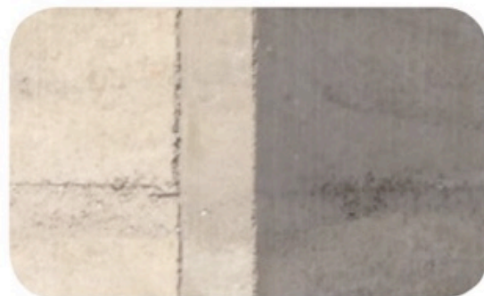
Rammed earth wall. Light in colour
